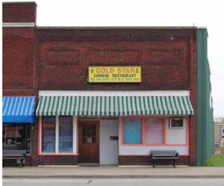
Photo of Existing Façade
