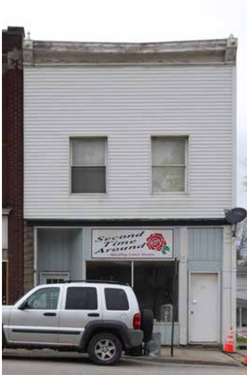
Photo of Existing Façade
