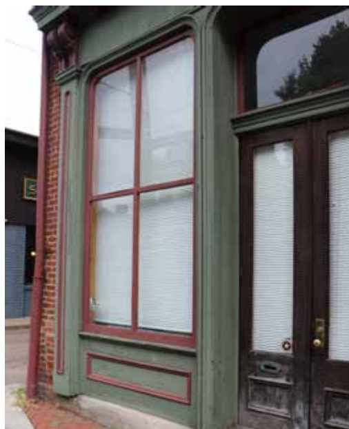
Historic Storefront Window
