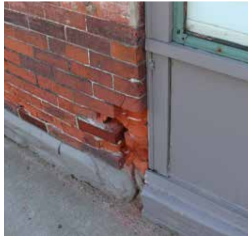
Photo of Side Window and Masonry Connection
