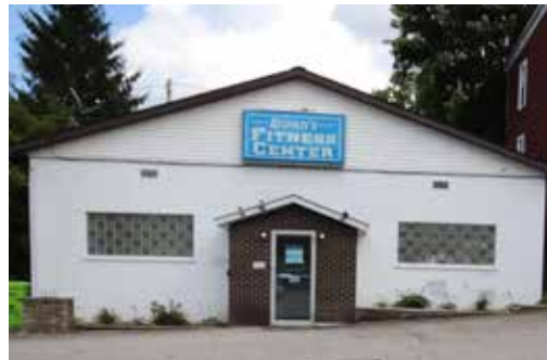
Gable Roof on the building at 1 South Main Street
