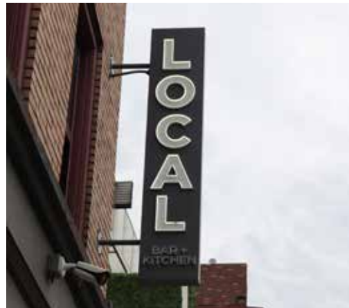
Appropriate internally illuminated projected sign
