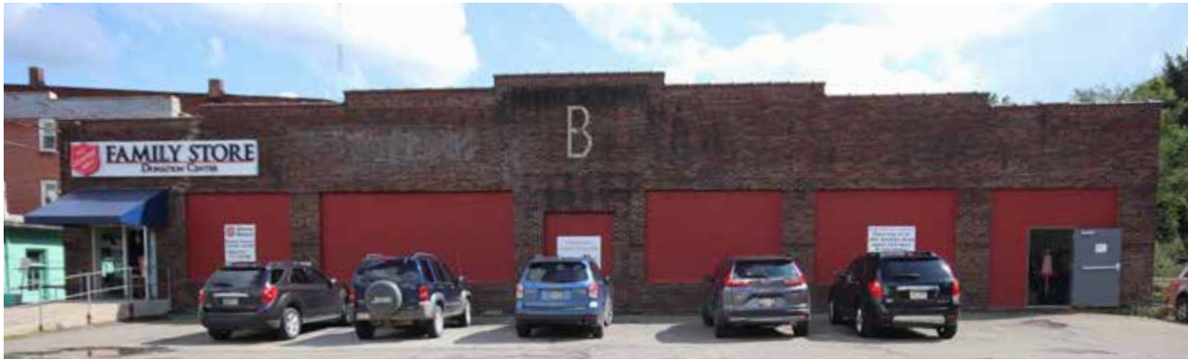
Photo of Existing Façade
