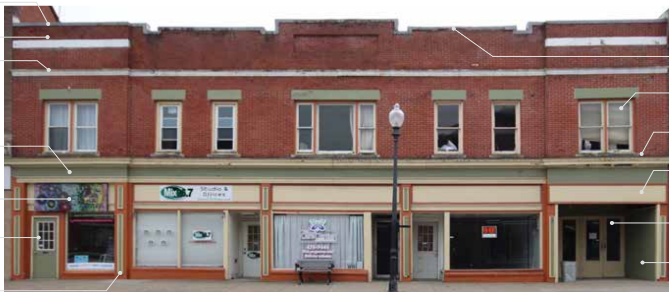
Photo of Existing Façade
