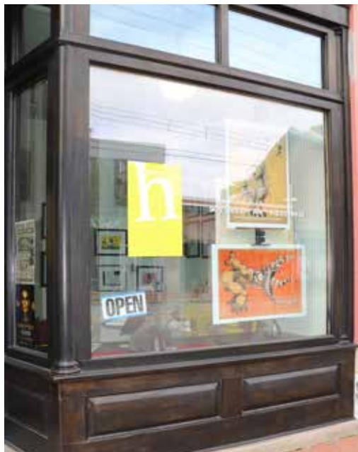
New Storefront has appropriately sized display windows and transoms
