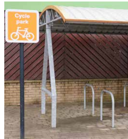
Covered Bicycle Parking shelters bicycles for long-term parking or during heavy rains
