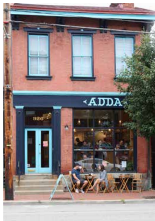
Historic Double-Hung Windows on upper floor with appropriate modern storefront windows
