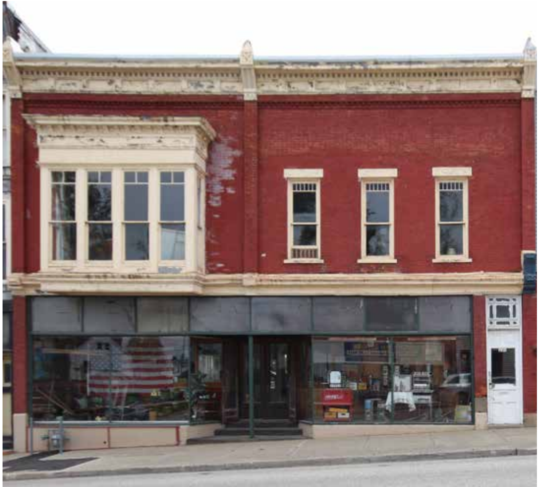
Photo of Existing Façade
