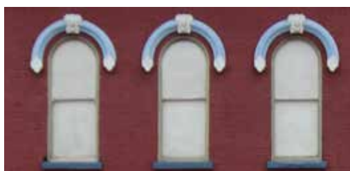
Arched Double-Hung Window 1/1 (one pane over one pane)
