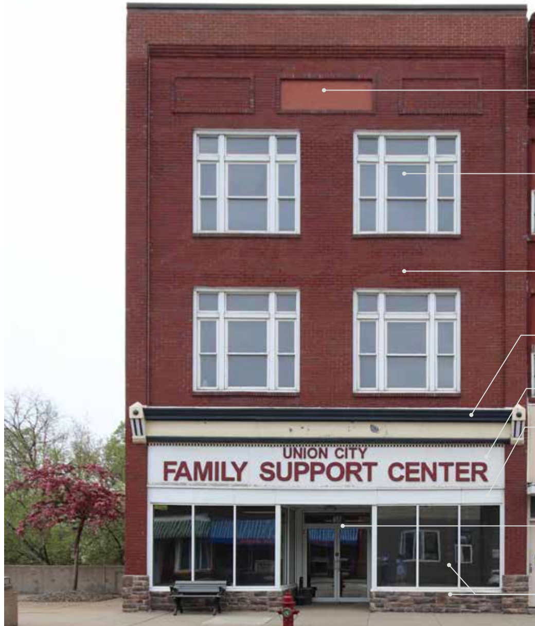
Photo of Existing Façade
