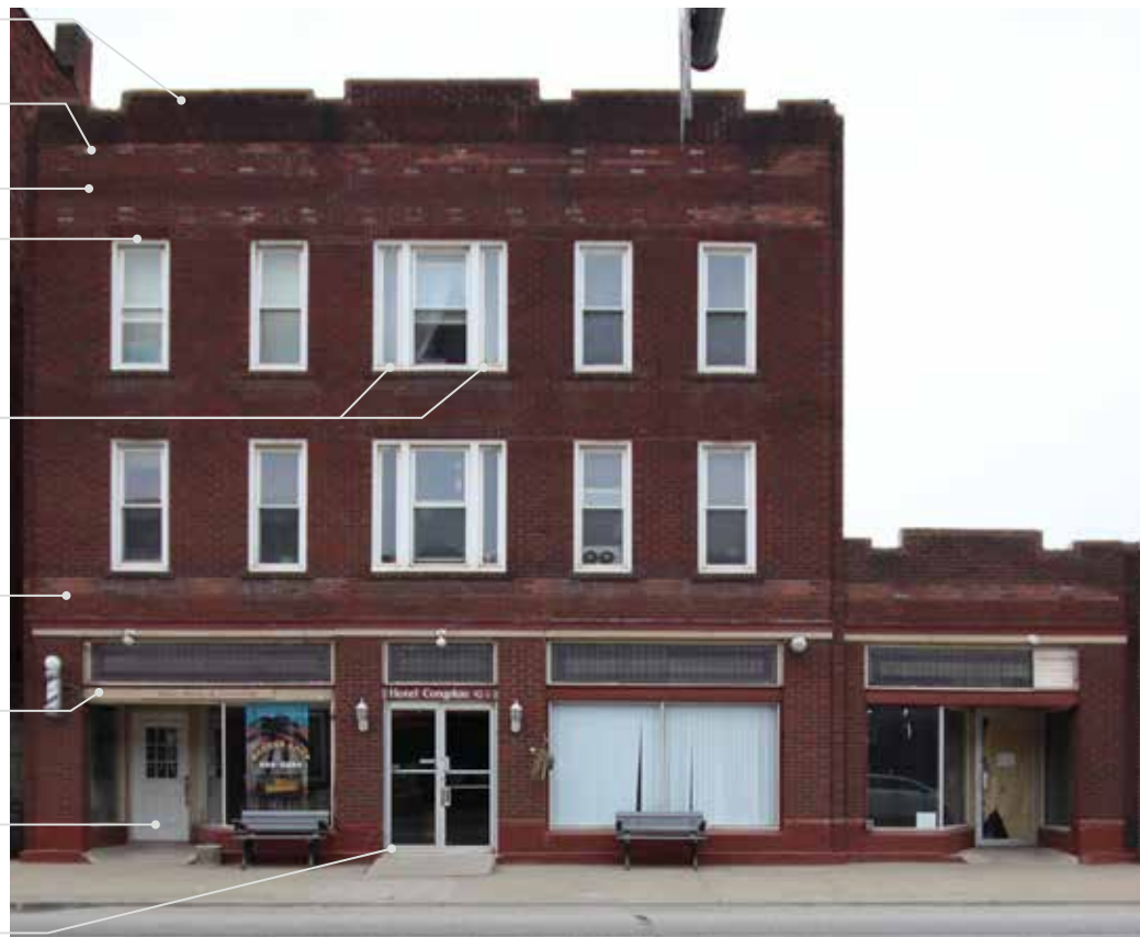
Photo of Existing Façade
