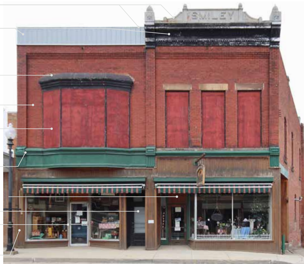
Photo of Existing Front Façade
