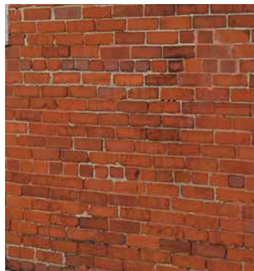
Masonry should be repointed every 15-30 years
