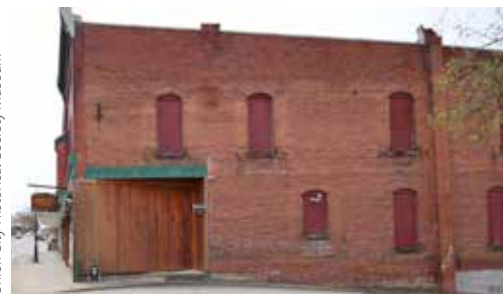
Photo of Existing Side Façade
