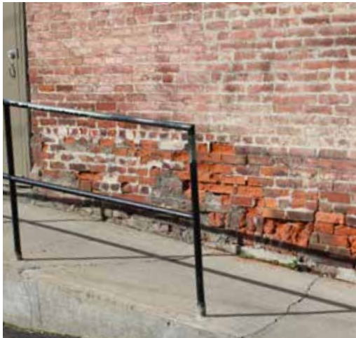
Photo of Rear Masonry Wall
