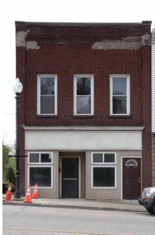
Photo of Existing Façade
