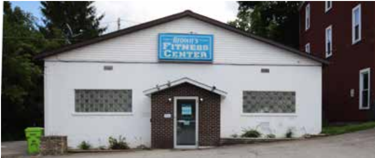
Photo of Existing Façade
