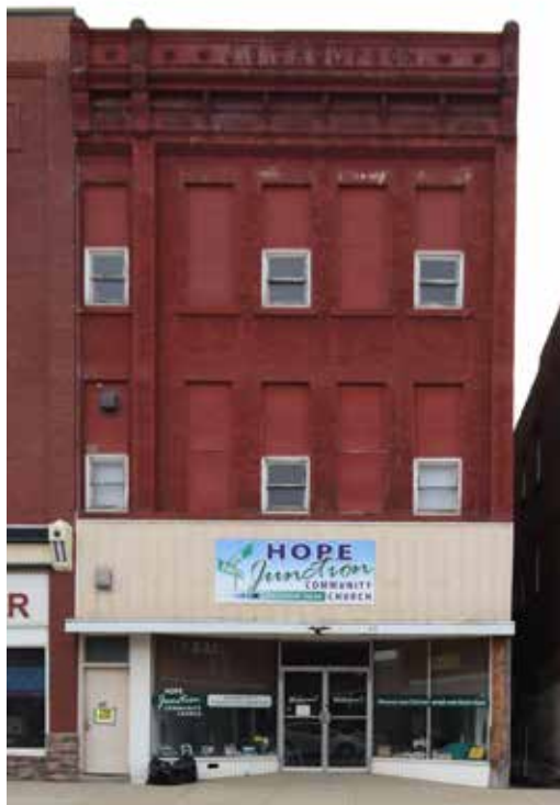
Photo of Existing Façade
