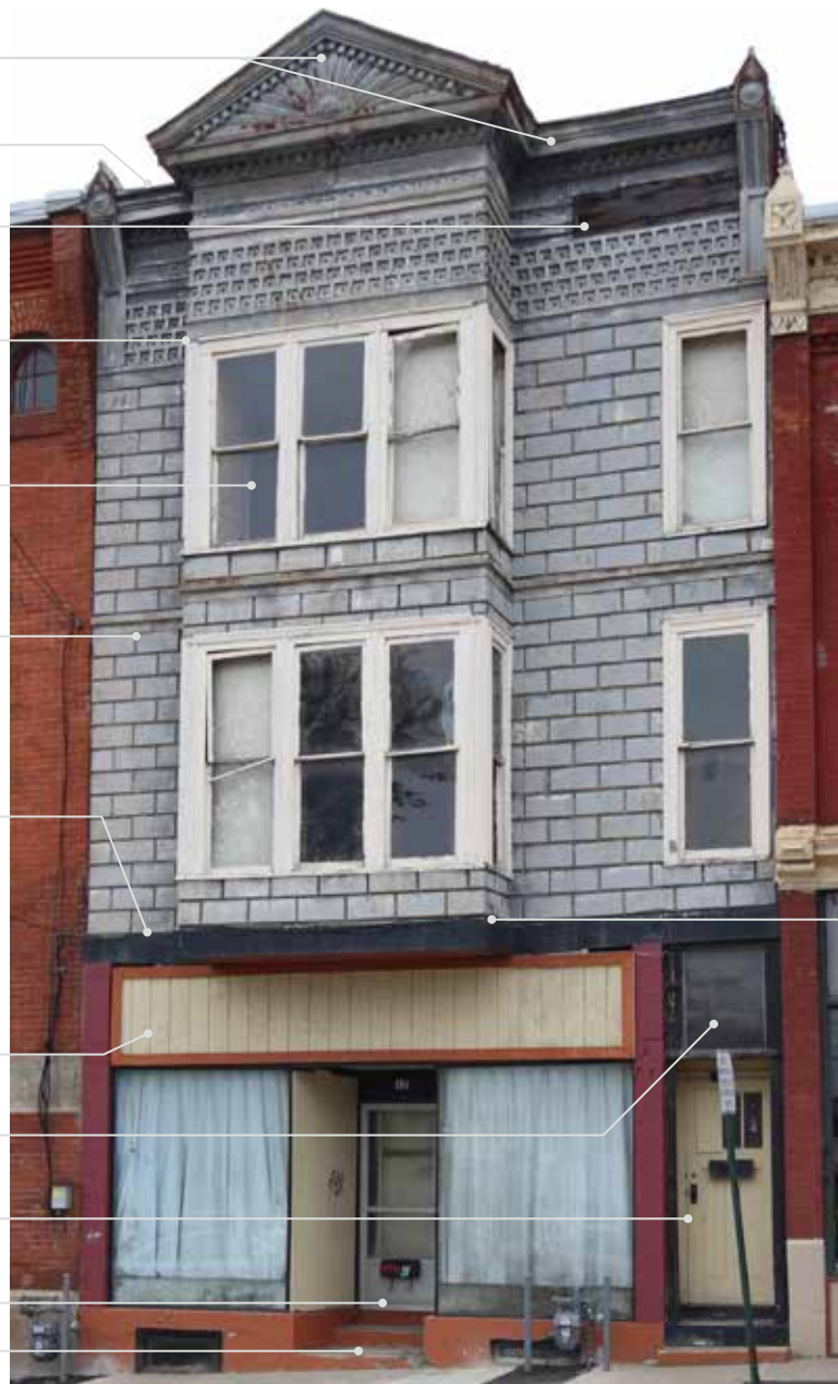
Photo of Existing Façade
