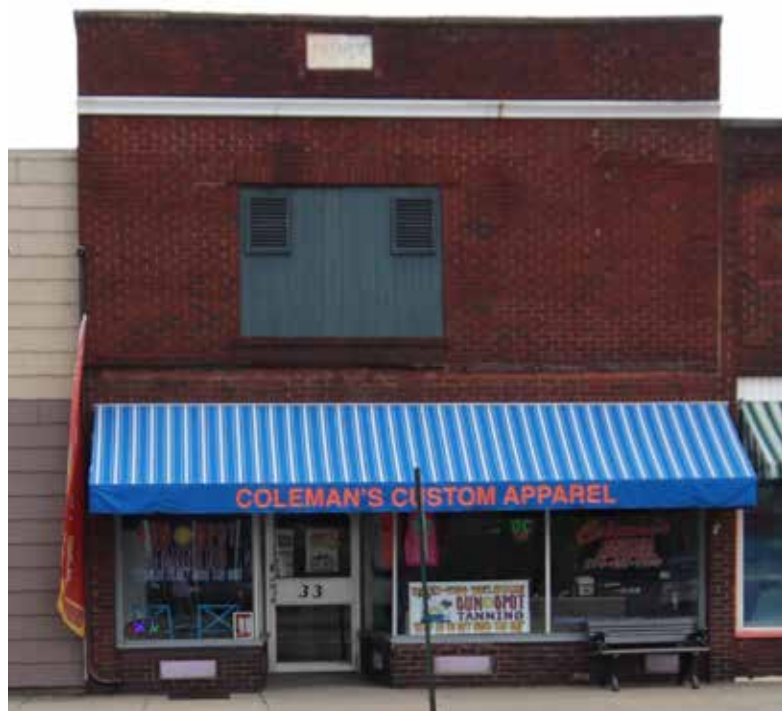
Photo of Existing Façade
