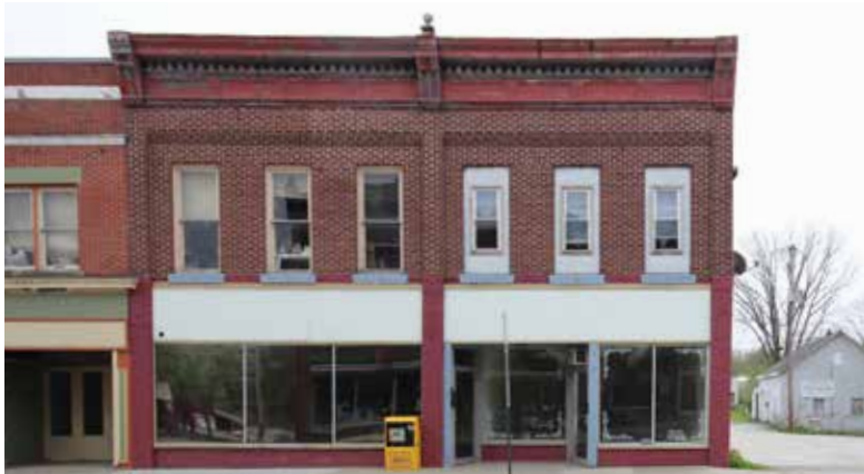
Photo of Existing Façade
