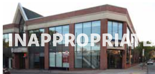
Inappropriate Fenestration does not blend with adjacent buildings. Often the window and door openings are too large or too little in comparison to surrounding historic buildings. In addition, the openings can appear irregular and accidental, like the building in the right photo.
