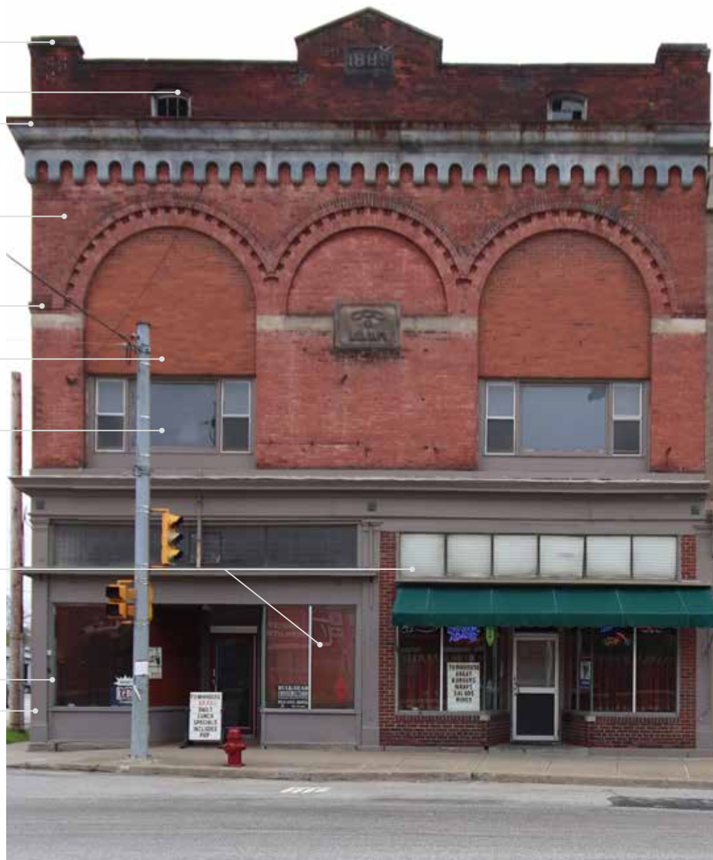
Photo of the Existing Main Street Façade
