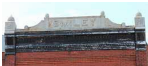
Metal Cornice maintain by painting, sealing and repairing flashing
