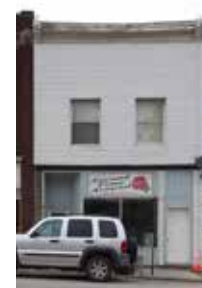
Photo of Existing Façade
