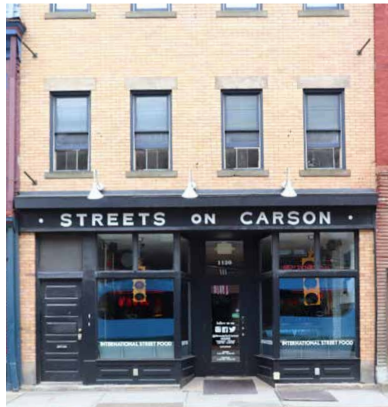
Gooseneck Light Fixtures located above the storefront and directed on the signboard
