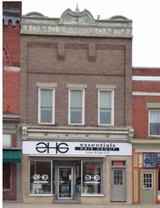
Photo of Existing Front Façade
