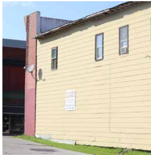
Gable Roof with Front Parapet on the building at 5-7 North Main Street
