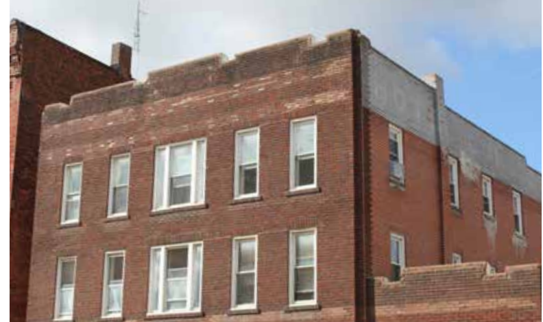
Low Slope Parapet Roof at 42 North Main Street
