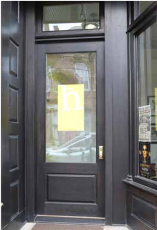
New Wood Storefront Door has historic details and proportions
