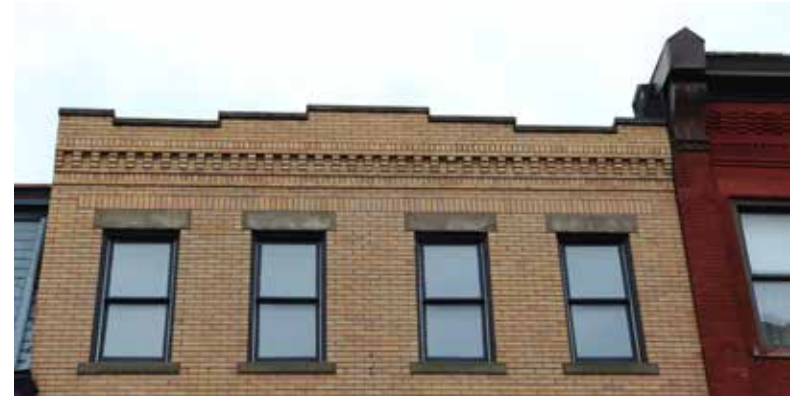
Low Slope Parapet roof with corbeled brick and stone cap
